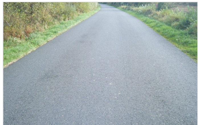
Road Mesh was installed in 2003
