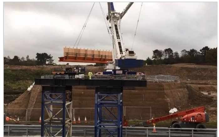
View of the Green Terramesh® slope
