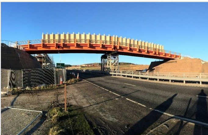
24m span bridge with bank seats directly over the Great Tower at the site
