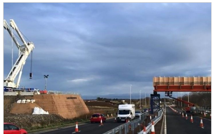
View of the Green Terramesh® slope
