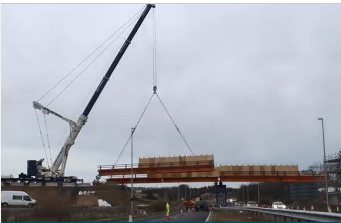
Heavy lifting crane supported by the Green Towers at the site
