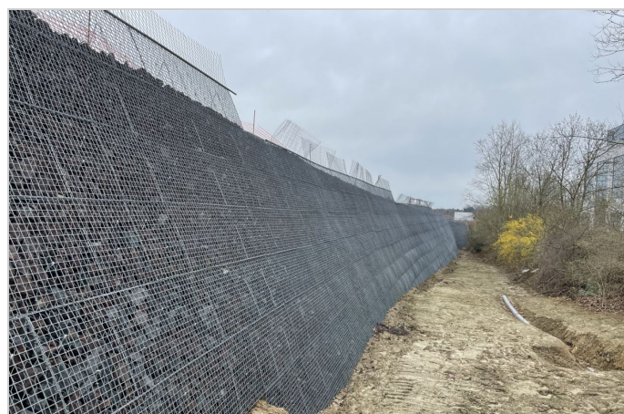
End of installation of MTM units
