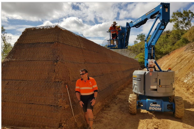
GTM embankment: Workers on EWP filling top most level of GTM cage
