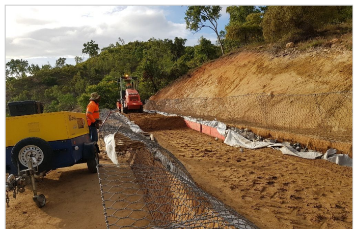
GTM embankment: Compaction of fill in progress
