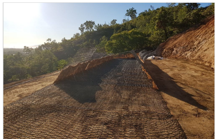
GTM embankment: Fixing of GTM lowest cage in progress
