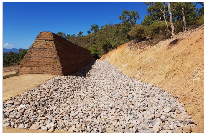
GTM embankment: complete installation (upslope view)
