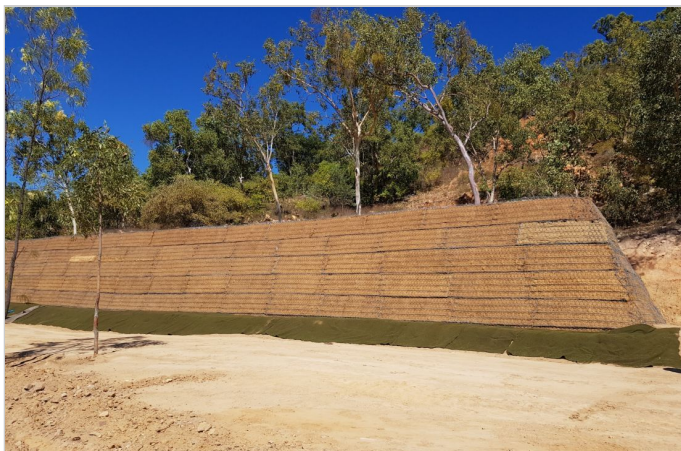
GTM embankment: complete installation (downslope view)
