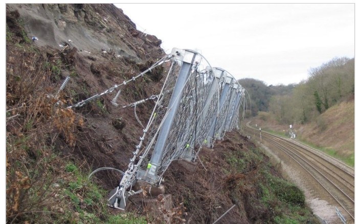
Barrier / Catch fence above railway line
