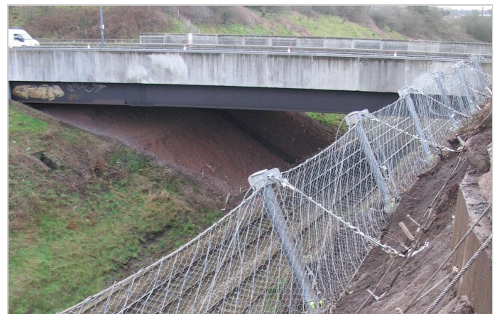
OM250 barrier installed above the Bristol - London railway line
