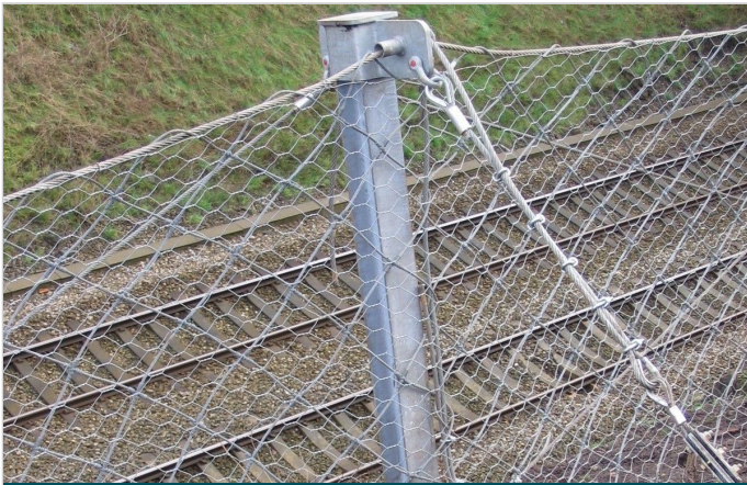
Intermediate fence post head detail
