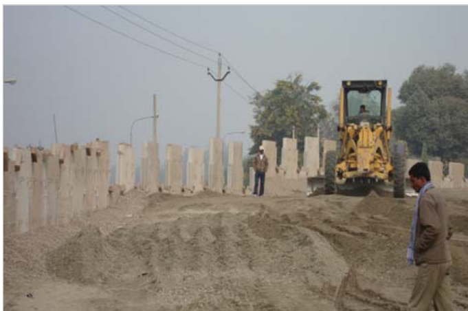
Photo 3: Construction of RS wall at curvature
