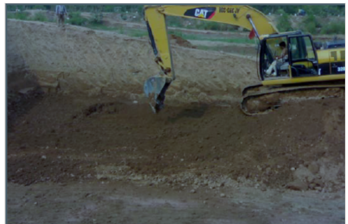
Photo 1: During construction— excavation
