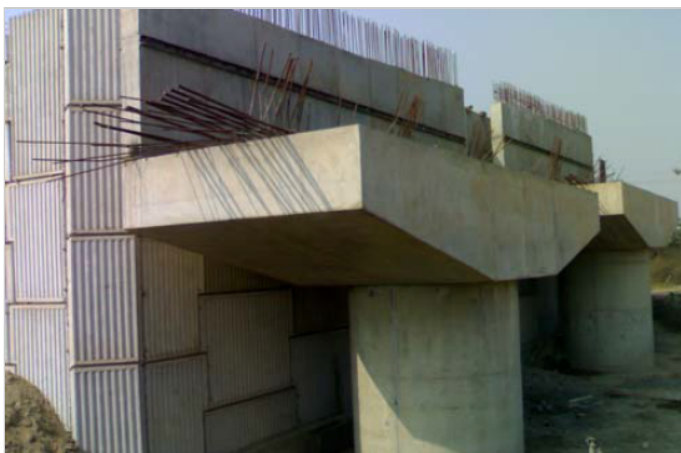
Photo 5: Closing RS wall near abutment
