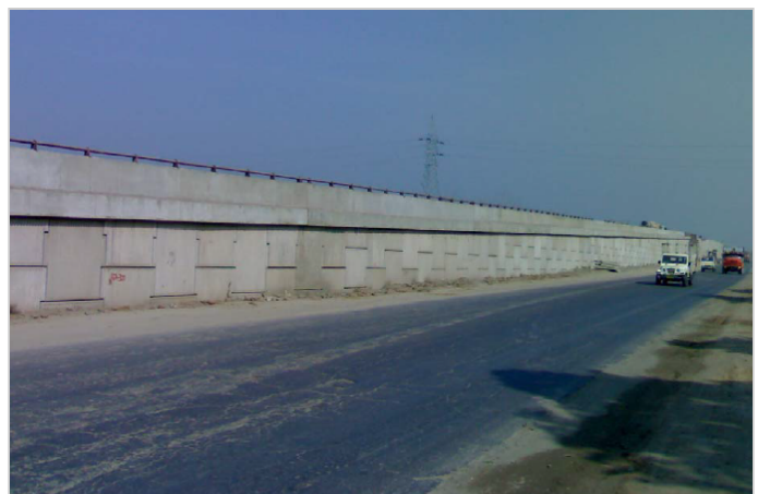
Photo 6: Complete approach ramp of RS wall
