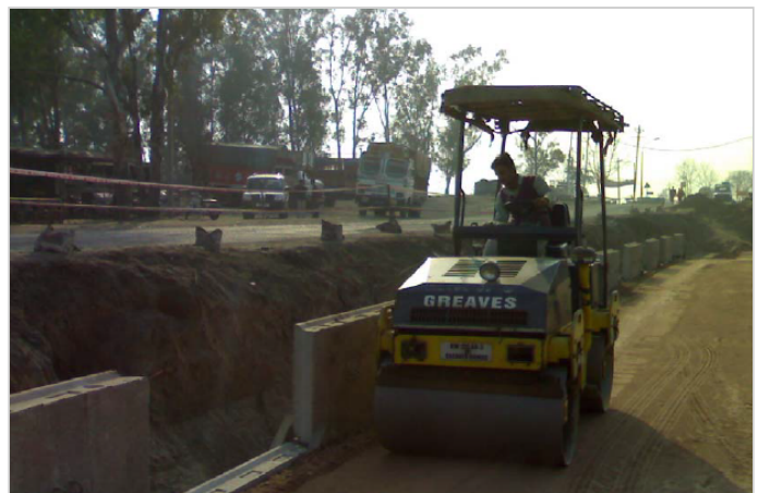
Photo 4: Compaction by baby roller in area close to wall
