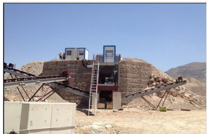
Terramesh System Retaining Wall
