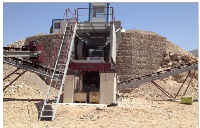
Terramesh System Retaining Wall
