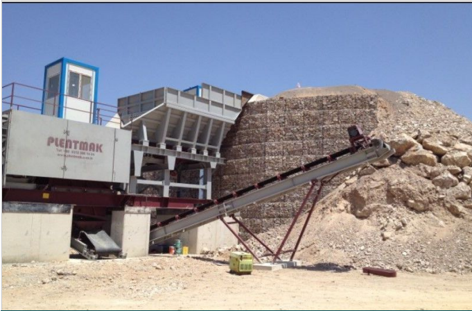
Terramesh System Retaining Wall
