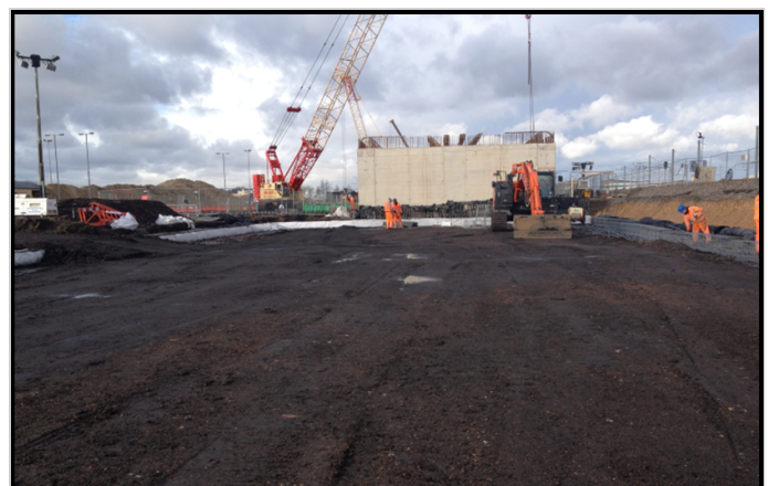
Compacted fill placed over Paralink LTP - April 2014
