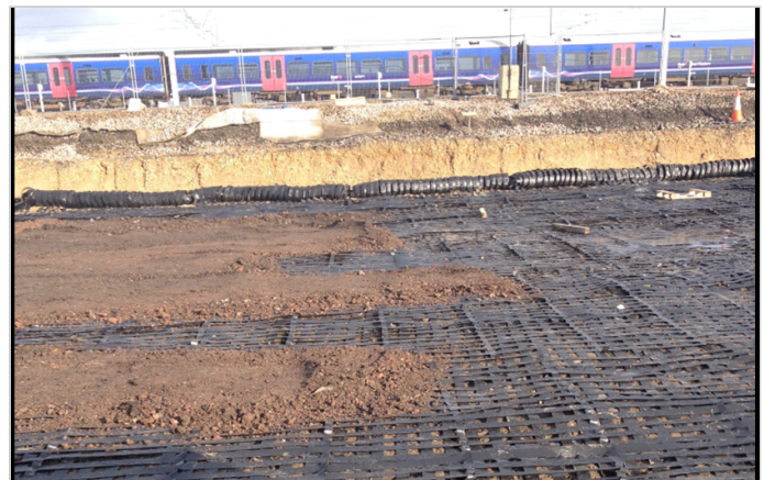
Load Transfer Platform with Paralink - March 2014
