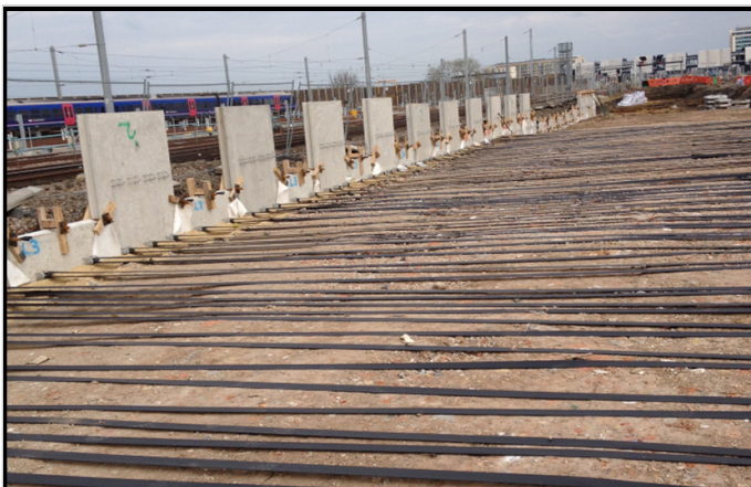
MacRes panels and Paraweb - East ramp during construction
