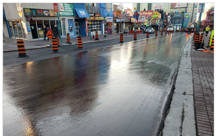
Tack coat application
