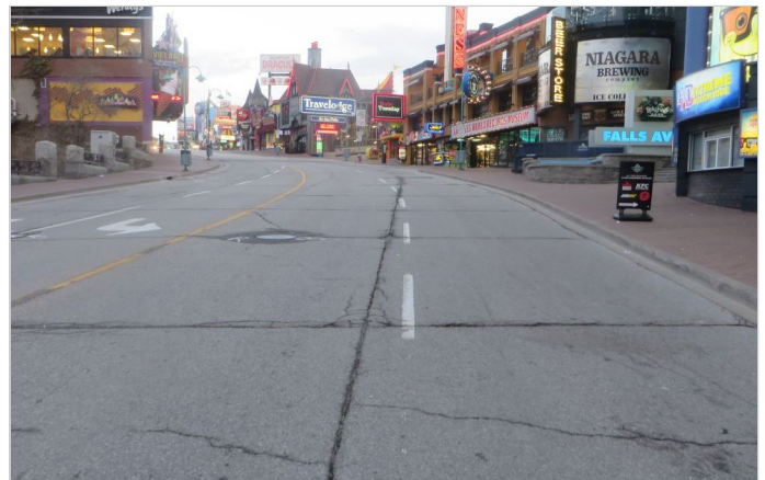
Pavement conditions before rehabilitation
