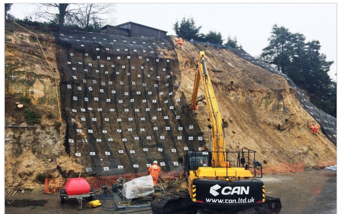
Preparing the netting along the rock face
