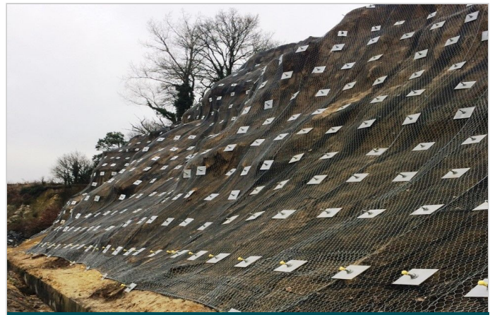
Securely nailed into the structure
