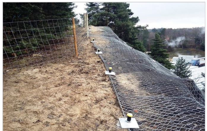
The top of the netting fastened by nailing into the soil
