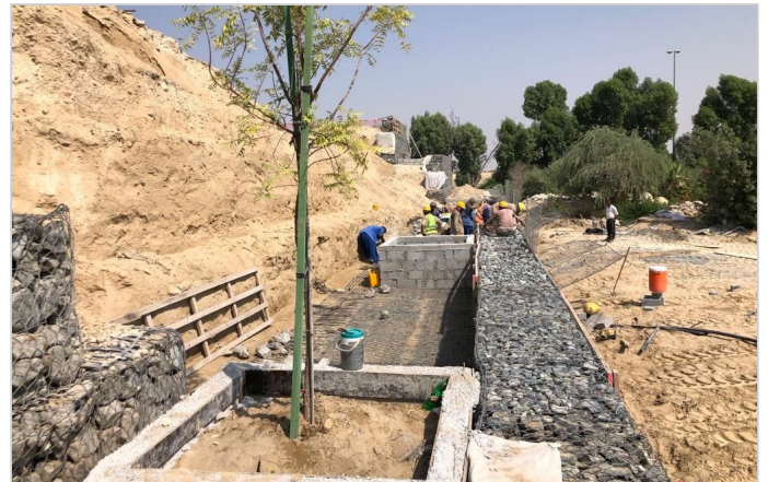
Terramesh MSE wall in progress
