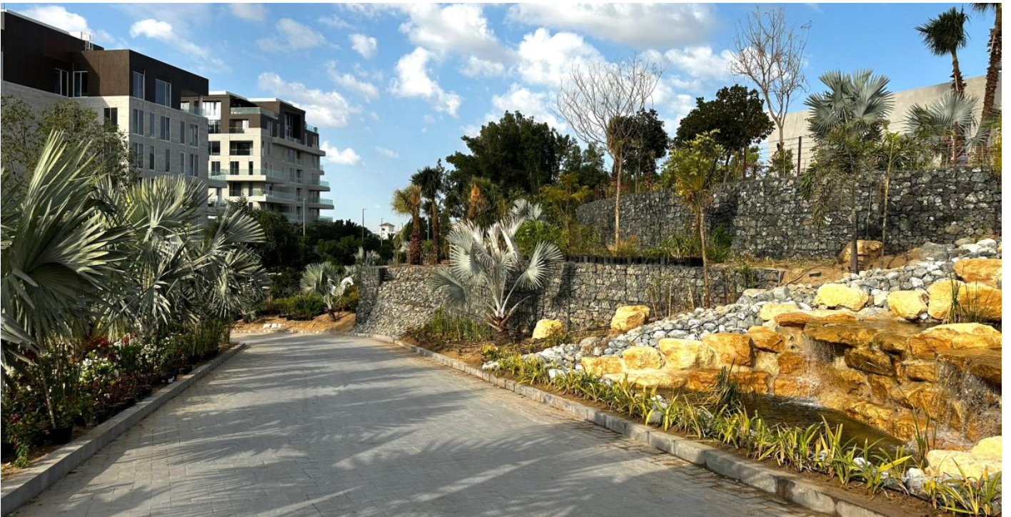
Completed Terramesh MSE wall with plantation works
