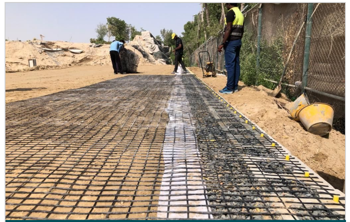
MacWall installation in progress
