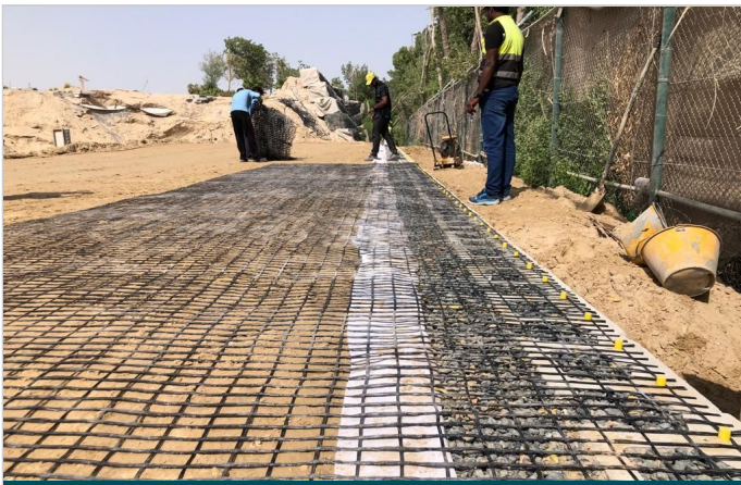
MacWall installation in progress
