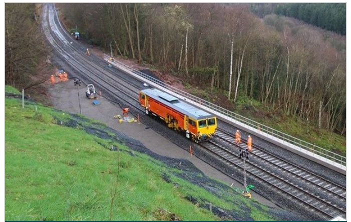
Works almost completed with 480m of new track installed
