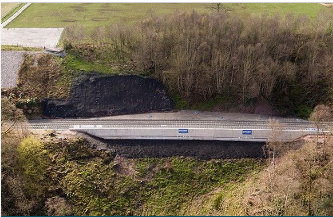
View of the site after the repair works
