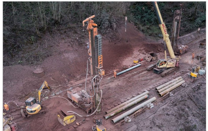
During construction in 2016
