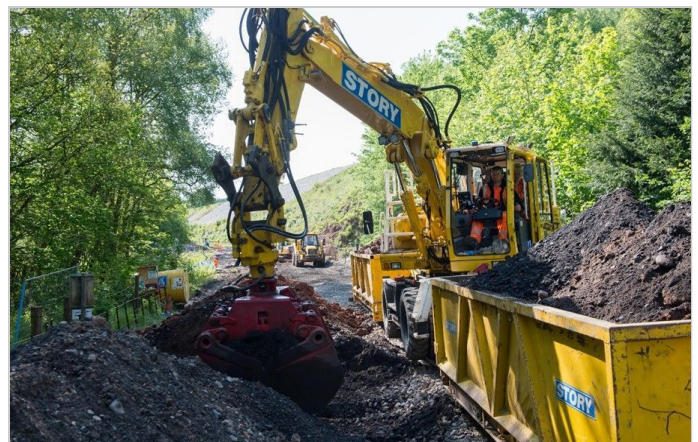
Story Contracting has removed 16,000 tonnes of soil from site
