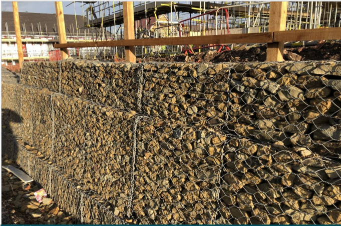
Gabion wall under construction
