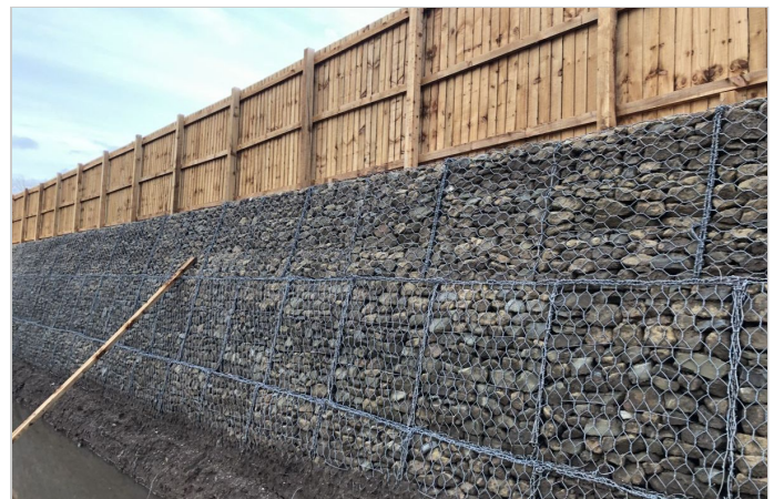
Finished gabion wall stretching along the line of properties
