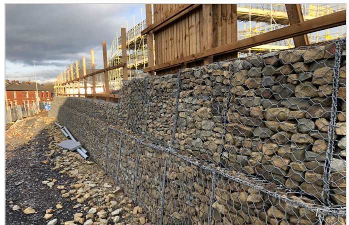
Gabion wall under construction
