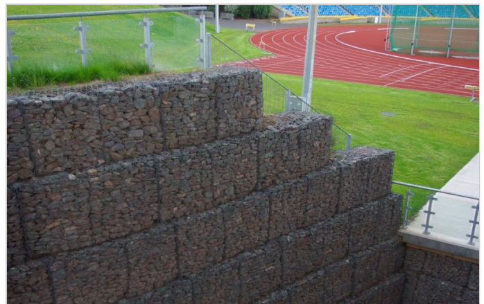
Completed Gabion Terramesh® wall
