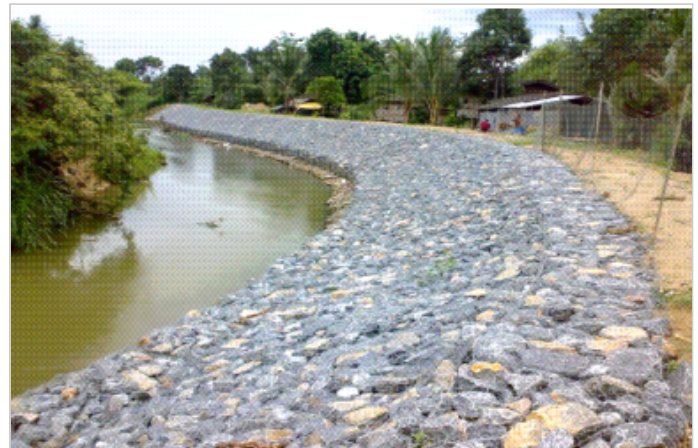
After construction (August 2008)
