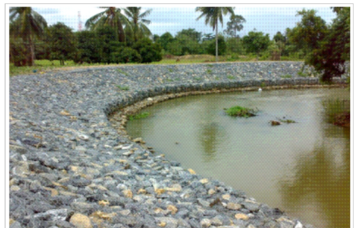
After construction (January 2008)
