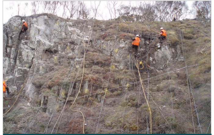
During construction using roped access specialists
