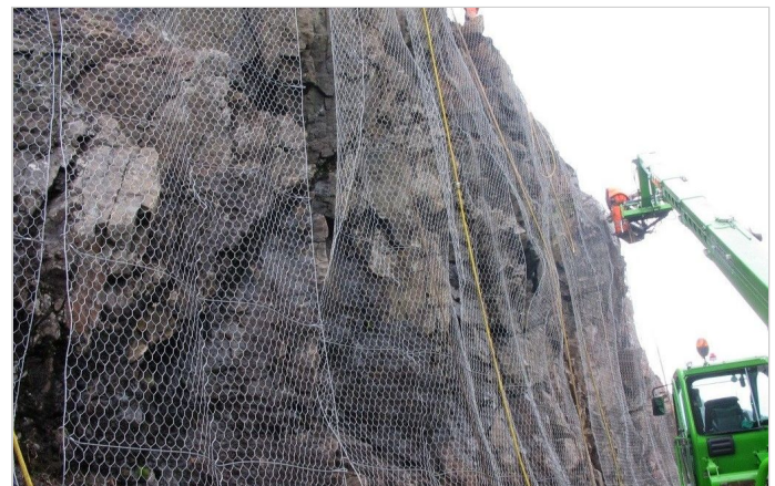
Hanging Steelgrid using trackside plant
