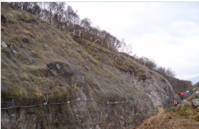
Project nearing completion
