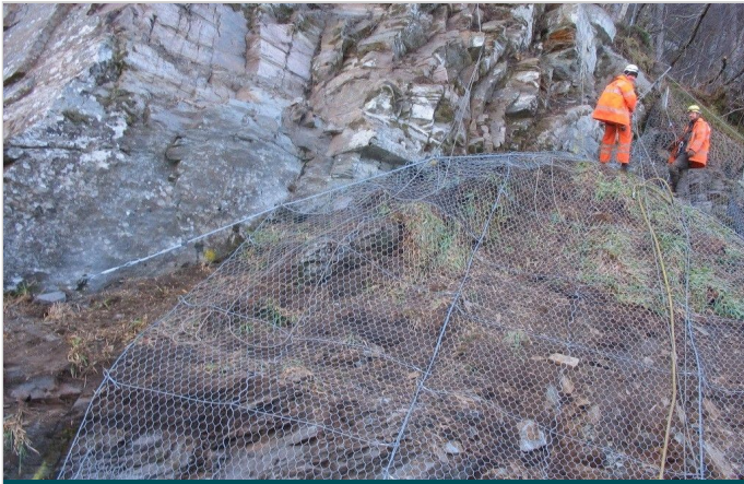
During construction using roped access specialists
