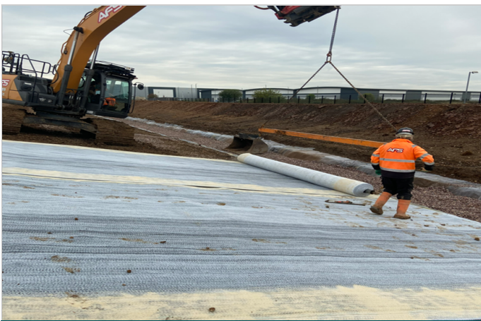
Bentonite powder is used to seal adjacent roll edges.
