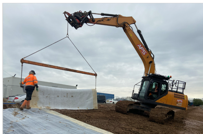
Macline GCL being installed with a spreader bar.
