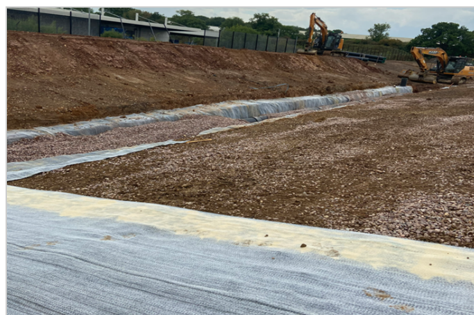
Macline GCL placed in drain trench to seal under filter drain.
