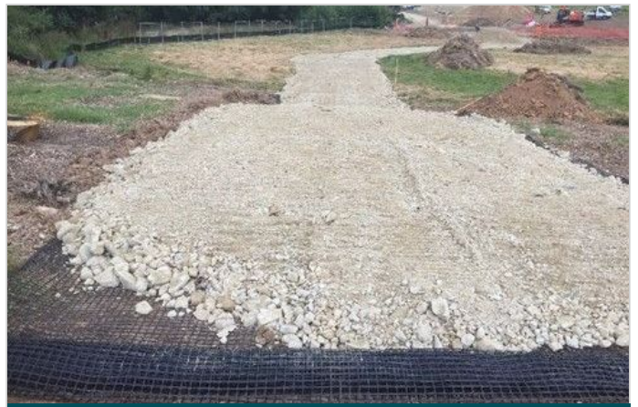
Macgrid WG S geogrids designed and installed for the
