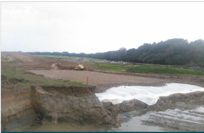
Mactex W2 (in white) installed over the soft clay sub
