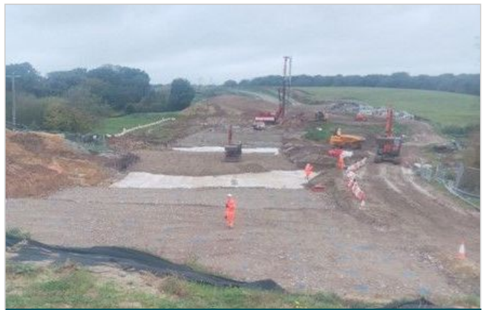
Working platform during the final stages of
