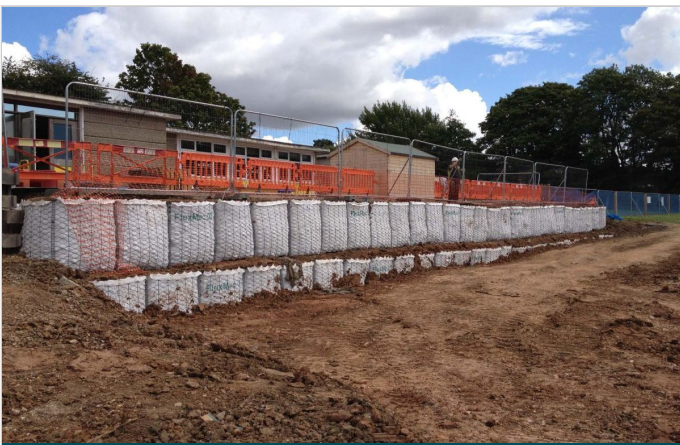
Completed temporary retaining structure, constructed in 2 days
