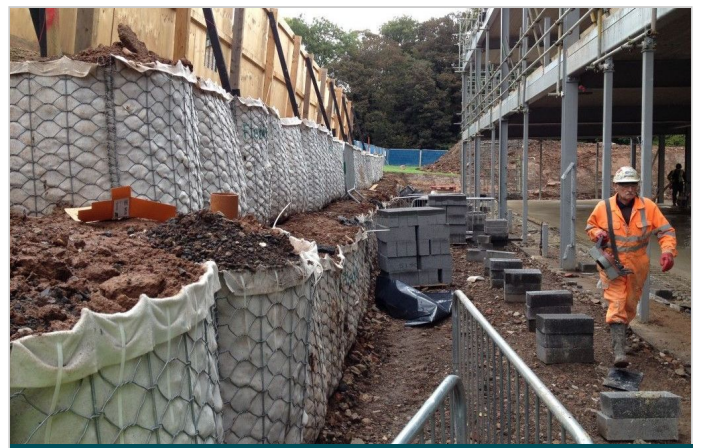
The completed temporary retaining wall following construction
