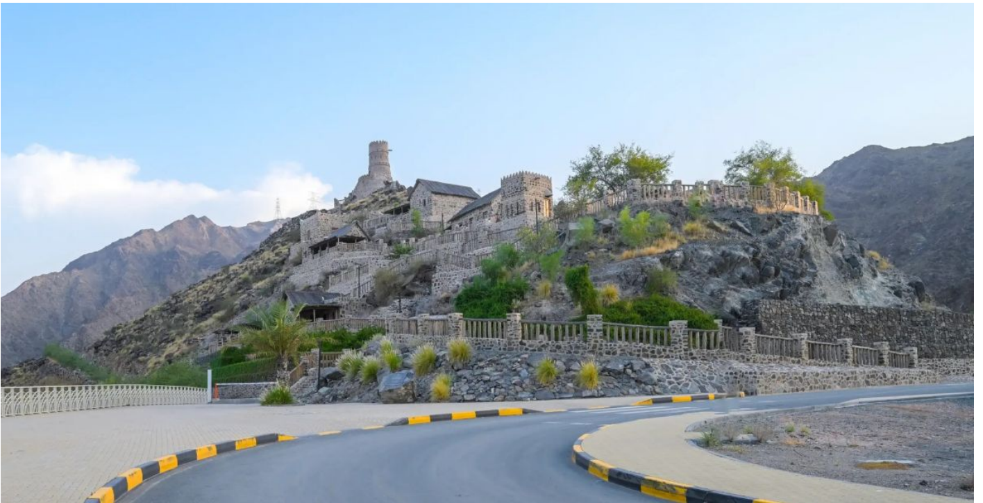
Completed Terramesh wall seamlessly integrated with the project site
