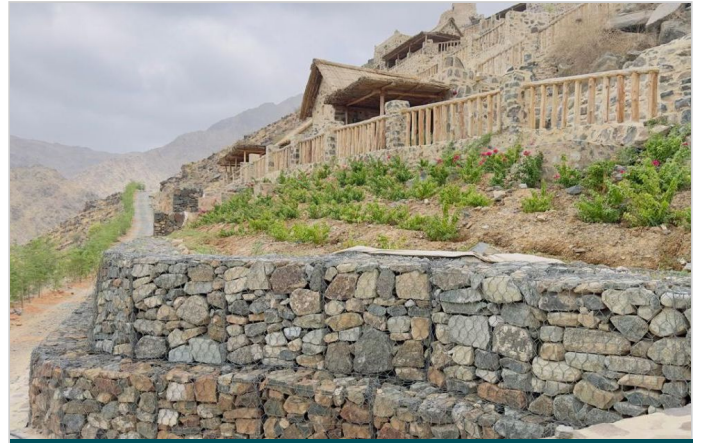
Completed wall: distant view
