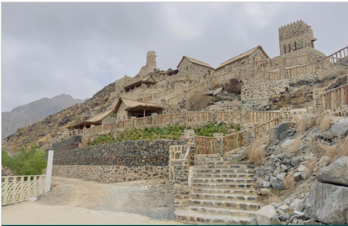
Completed wall: distant view
