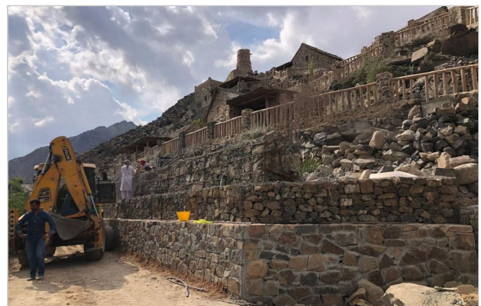
Terramesh wall in progress
