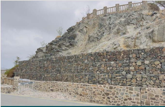
Completed wall: distant view
