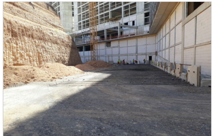
Precast Panel Retaining Wall - Polymer Stripes
