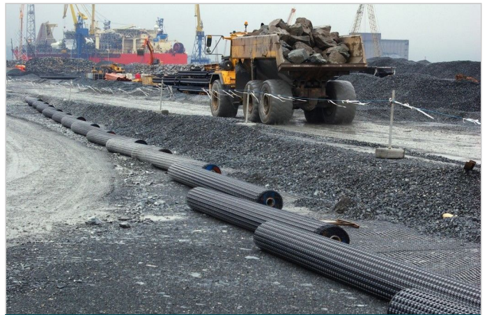
MacGrid laid on the upper layers of the pavement
