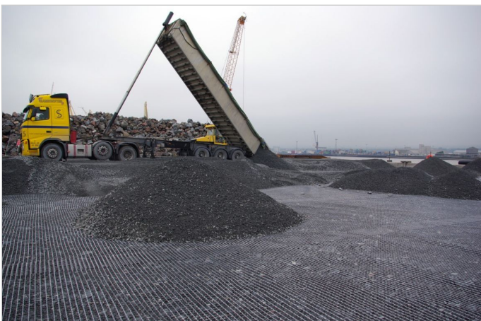
Granular material placed over MacGrid
