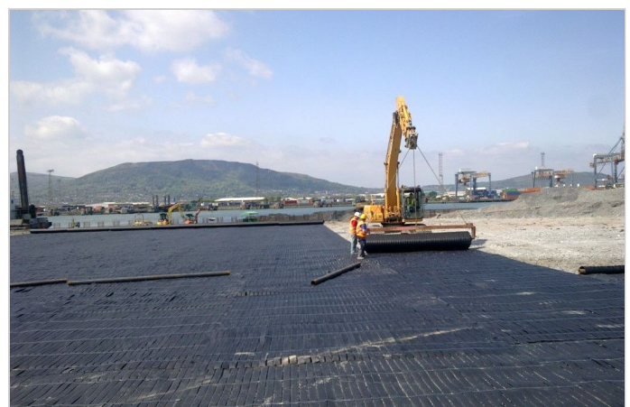
ParaLink® 1350 being laid
