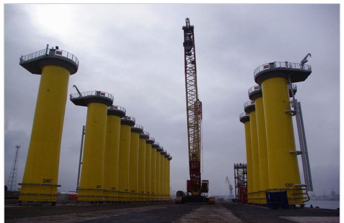
Heavy crane running over the reinforced ParaLink® pavement
