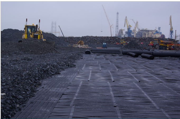
Filling granular material placed over ParaLink®
