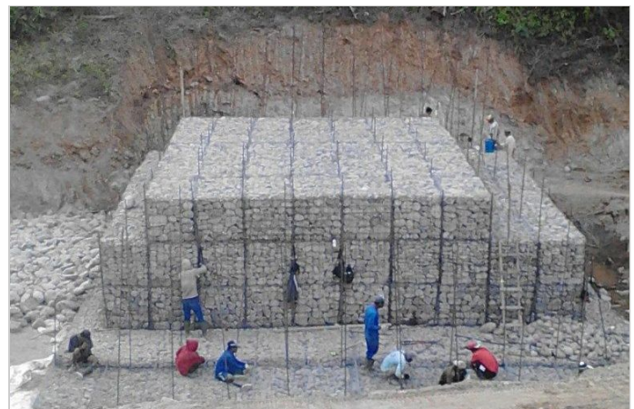
Weir Foundation Construction
