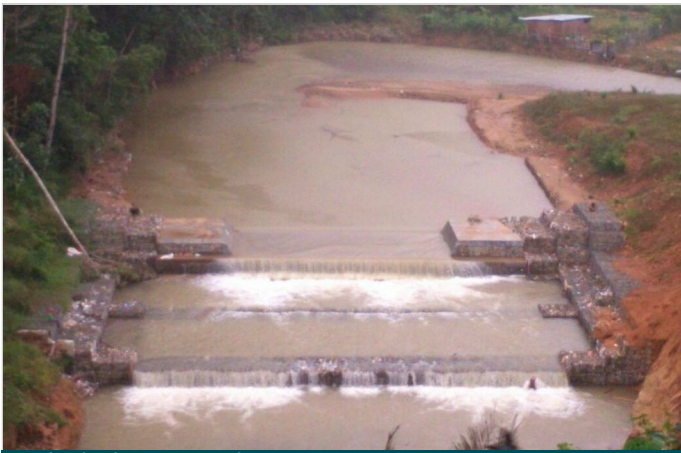
Weir during operation
