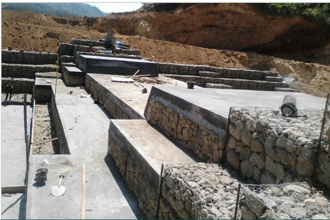
Gabion Concrete Capping
