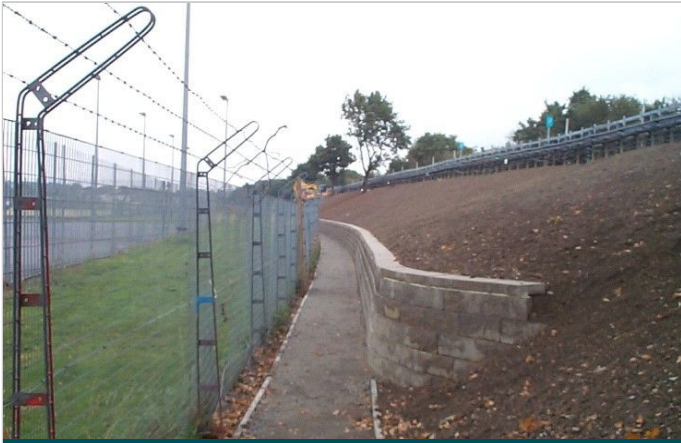
Post construction of MacWall
