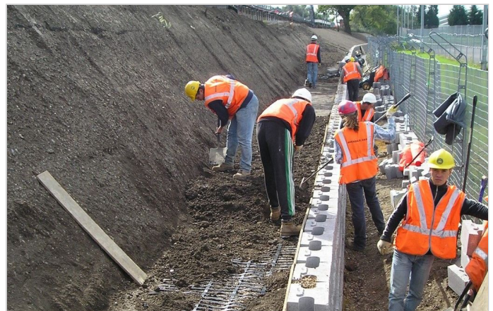
Construction of the MacWall Vertica
