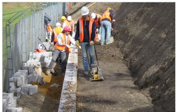
Post construction of MacWall
