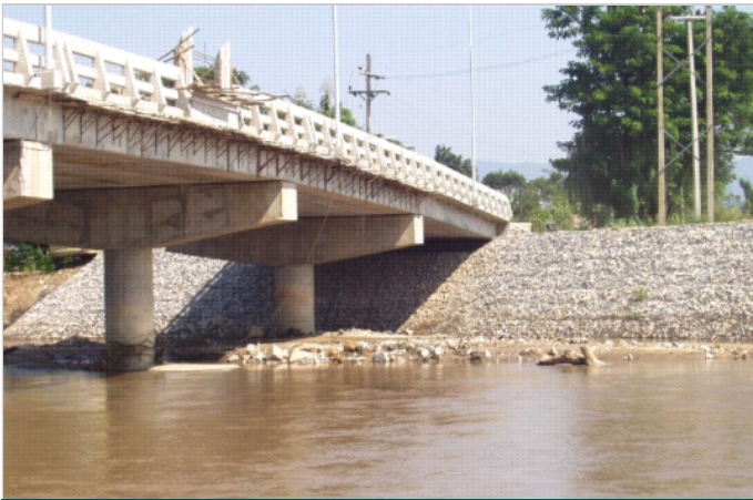
After construction (January 2008)
