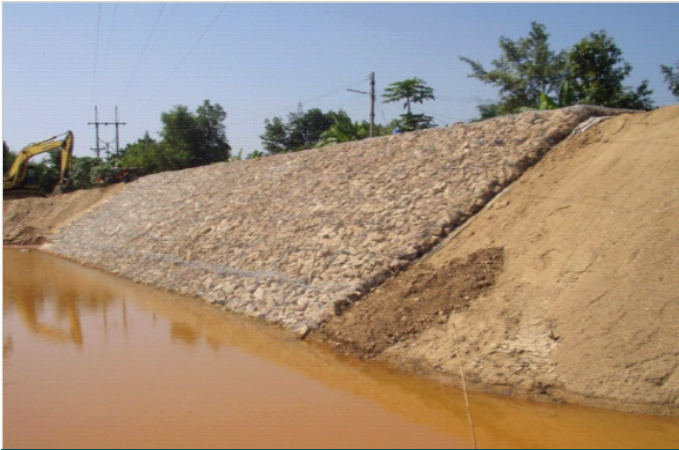
During construction (December 2007)
