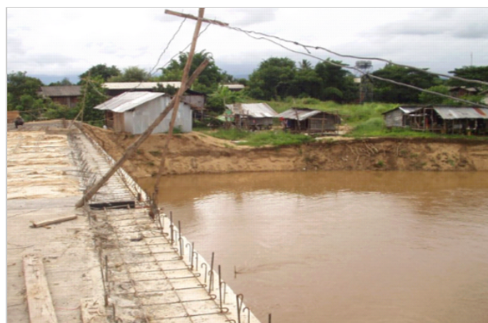
Before construction (October 2007)
