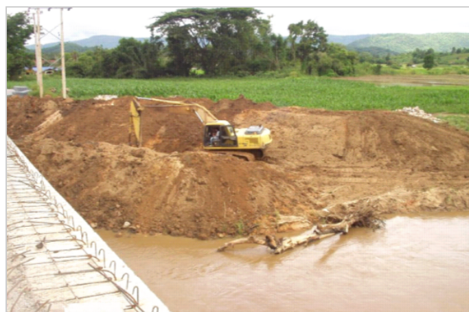
Durin construction (November 2007)
