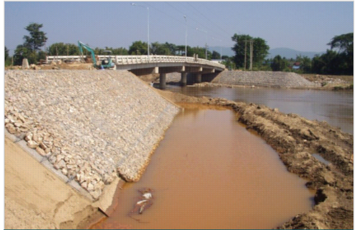
After construction (January 2008)
