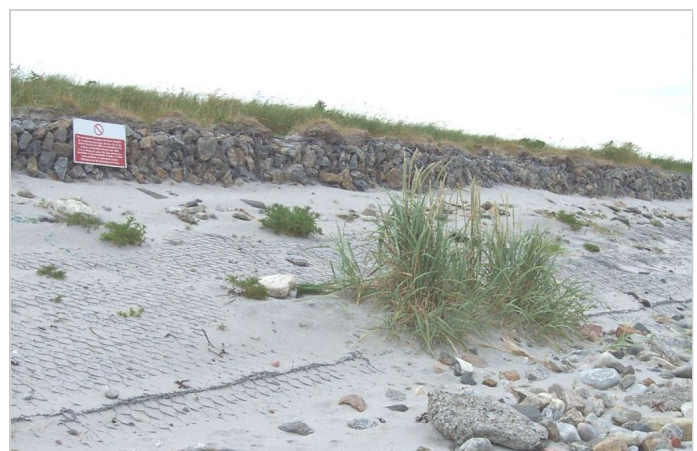
The revetment after construction - note accretion of sand
