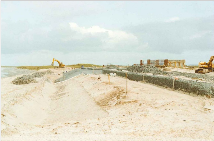
Construction on the airport slope
