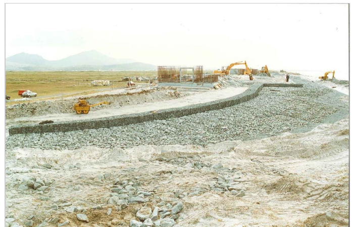
Original construction of revetment at firing range
