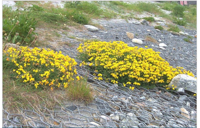
Vegetation establishing in revetment
