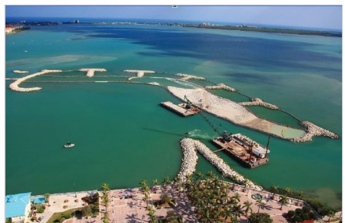
Islands Under Construction
