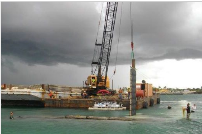
Maccaferri Polymeric Marine Mattress Installation
