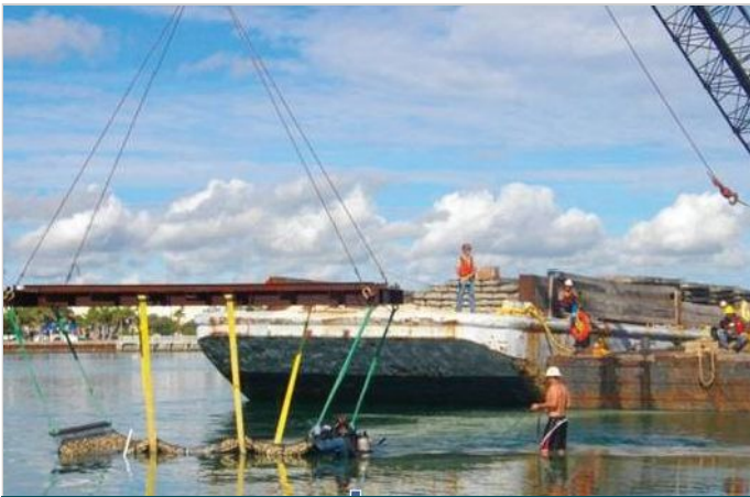
Maccaferri Polymeric Marine Mattress Installation
