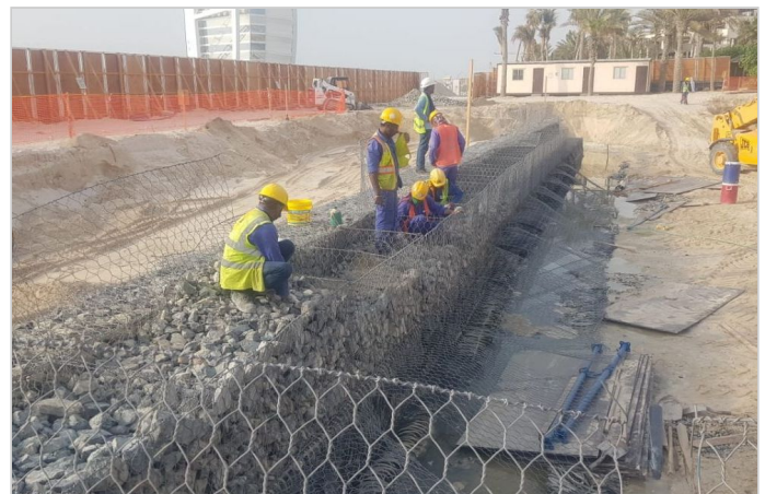
During construction: terramesh & Gabion protection walls in progress
