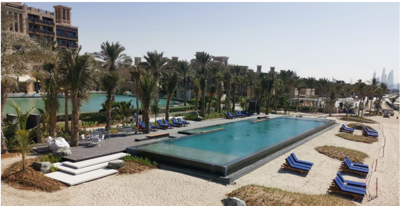
Distant view of completed pool constructed above buried protection structures
