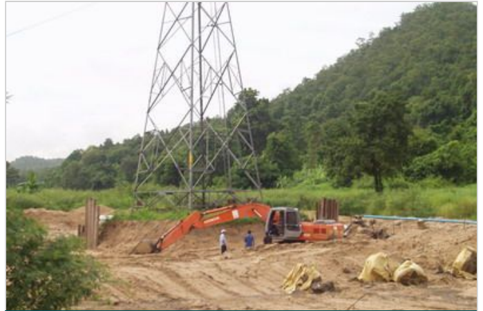
Gabion wall construction (4)
