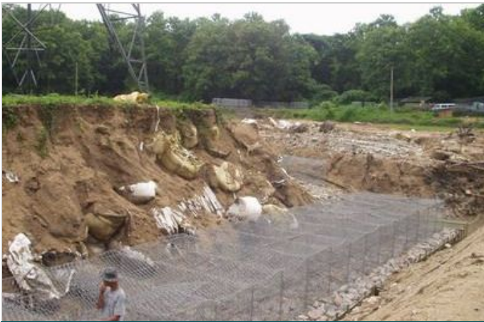
Gabion wall construction (5)
