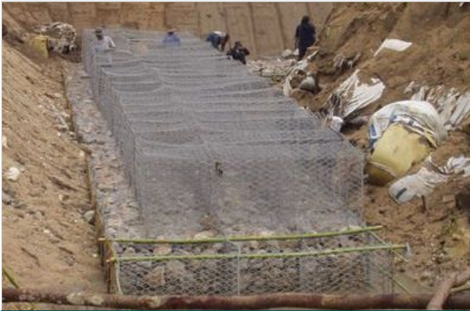
Gabion wall construction (3)
