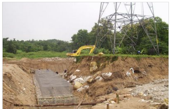
Gabion wall construction (1)
