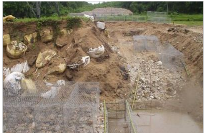
Gabion wall construction (6)
