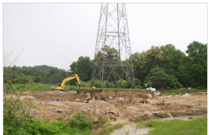
Gabion wall construction (2)
