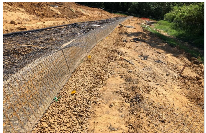
Green Terramesh unit erected - no external formwork needed
