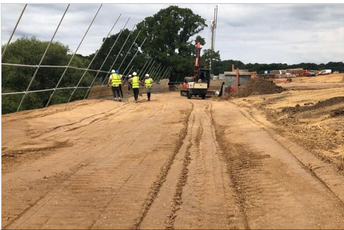
Lime treated backfill placed and compacted
