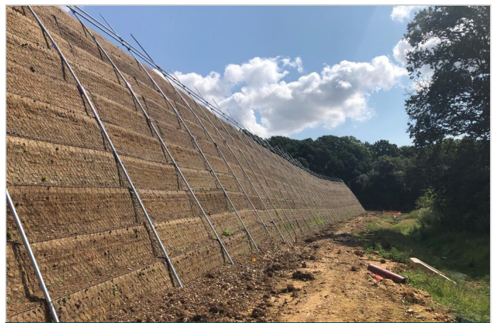
Green Terramesh slope gaining height - note edge protection
