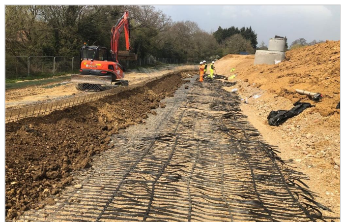
ParaGrid placed ready for structural backfilling
