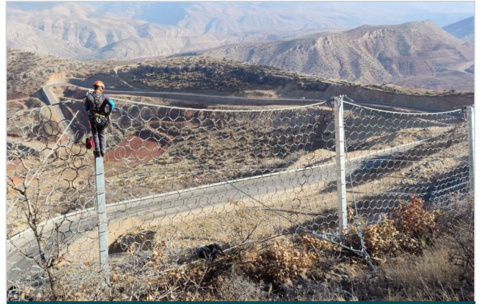
ROCKFALL BARRIER INSTALLATION
