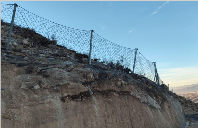
INSTALLED ROCKFALL BARRIER
