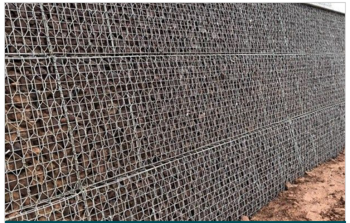
Mineral Terramesh during construction - face detail
