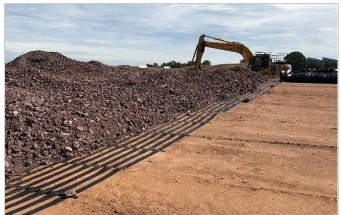
ParaLink basal reinforcement being installed
