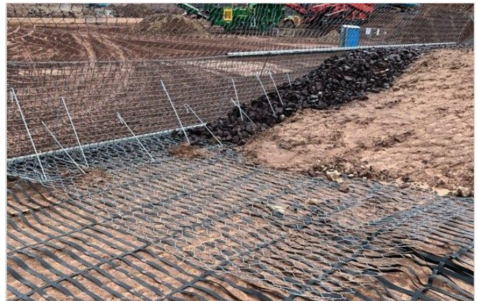
Mineral Terramesh bracing rods installed
