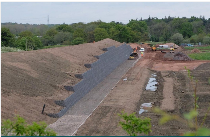
Mineral Terramesh structure reaching full height
