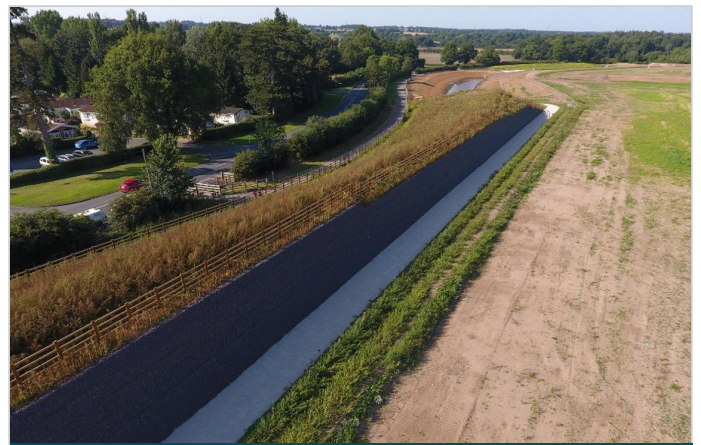
Completed Mineral Terramesh structure
