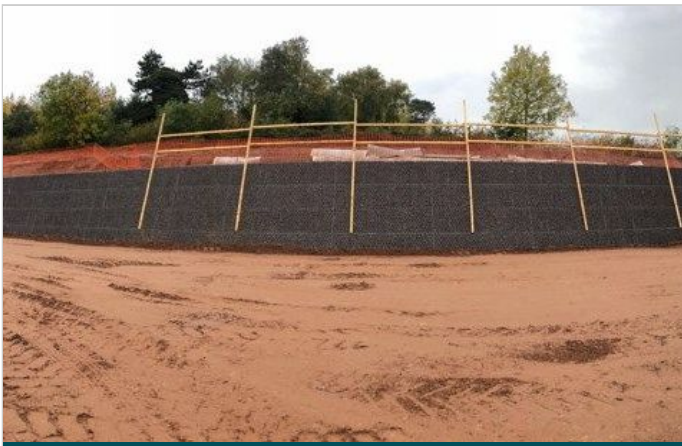
Eastern side bund Mineral Terramesh reinforced soil retaining wall
