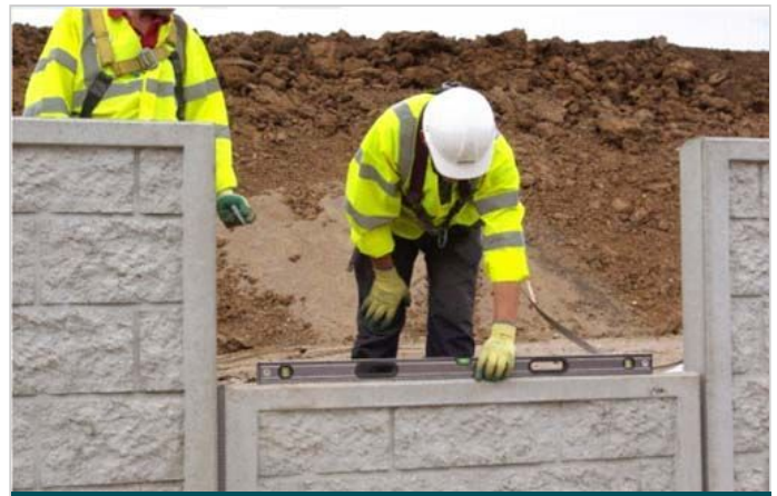
Checking line and level
