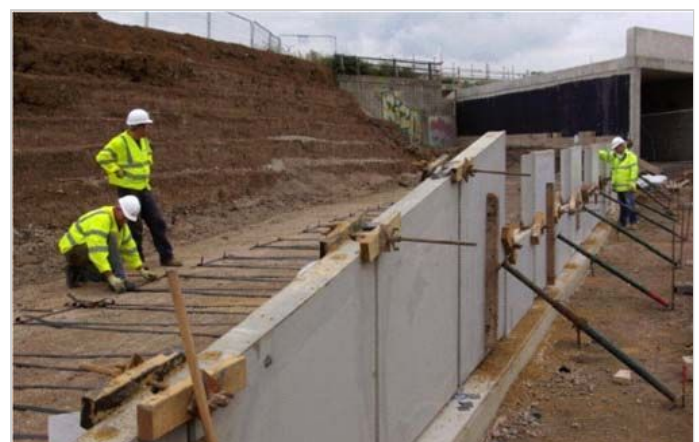
Propping face panels prior to backfilling
