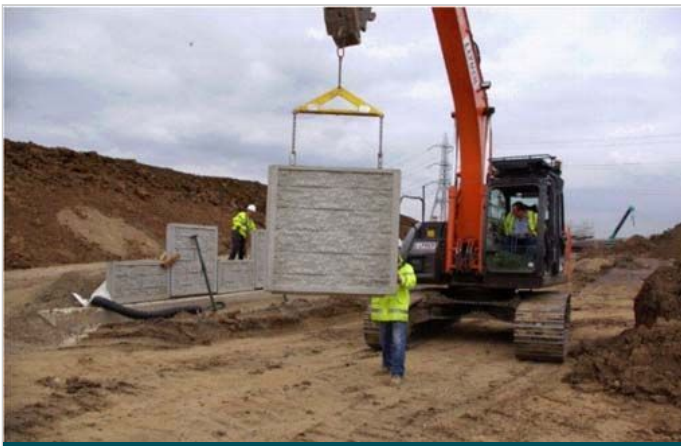
Lifting face panels into position
