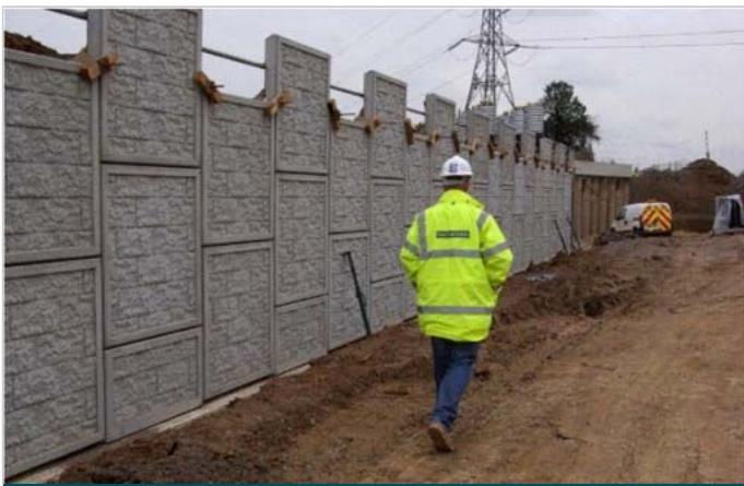
Panels ready for backfilling - note bespoke face finish
