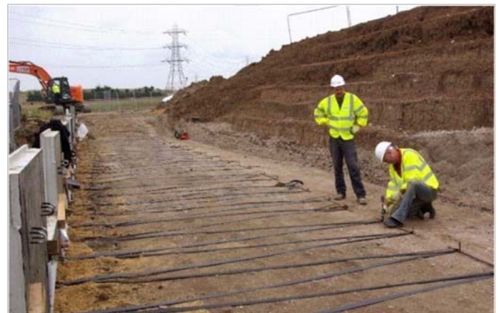
Placing & securing ParaWeb®
