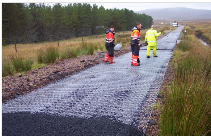
The B873 reconstructed with Road Mesh™
