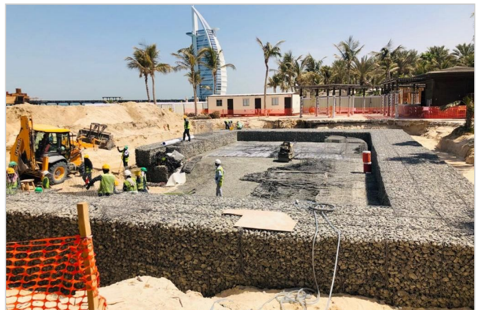
Terramesh System with Gabion sacrificial protection wall - during construction
