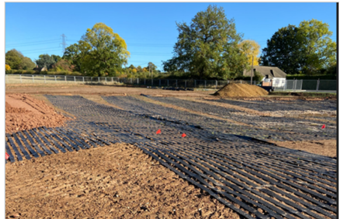
Paralink being installed within the embankment footprint.
