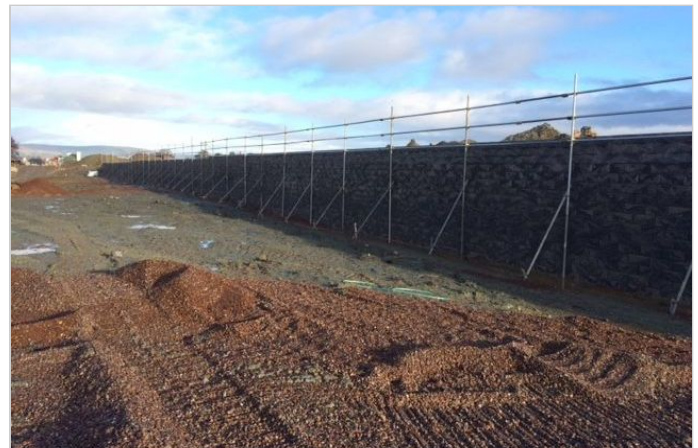
Construction of walls begin on site
