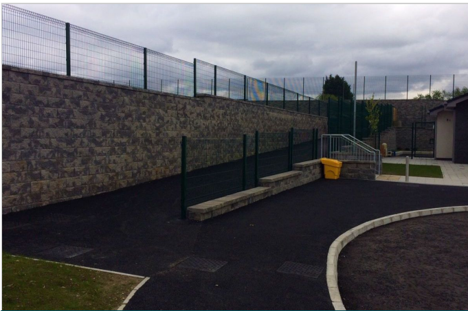
MacWall Vertica forming walkway
