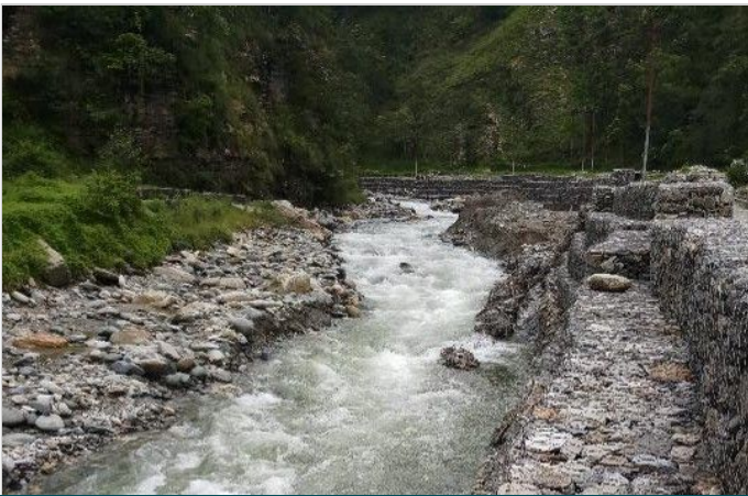
Photo 5: Completed protection work
