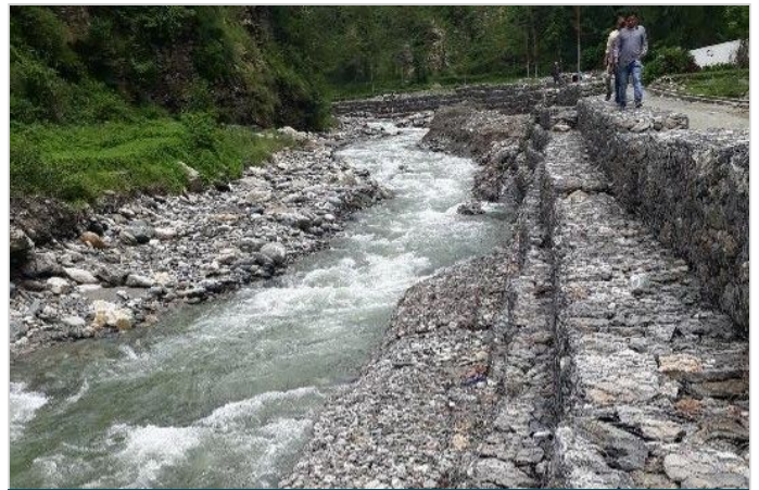
Photo 6: Completed protection work
