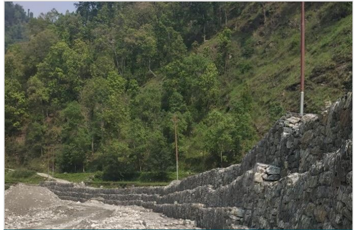
Photo 4: River bank protection / road embankment protection works
