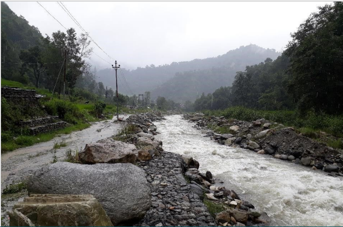
Photo 3: Initial site condition
