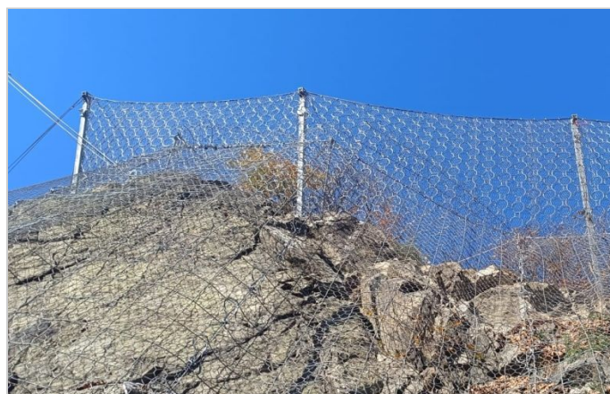
MacArmour & RB2000 installation
