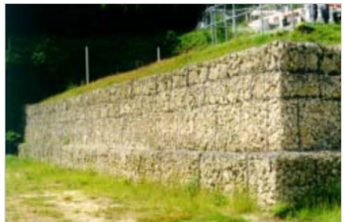
Front view of wall pre earthquake
