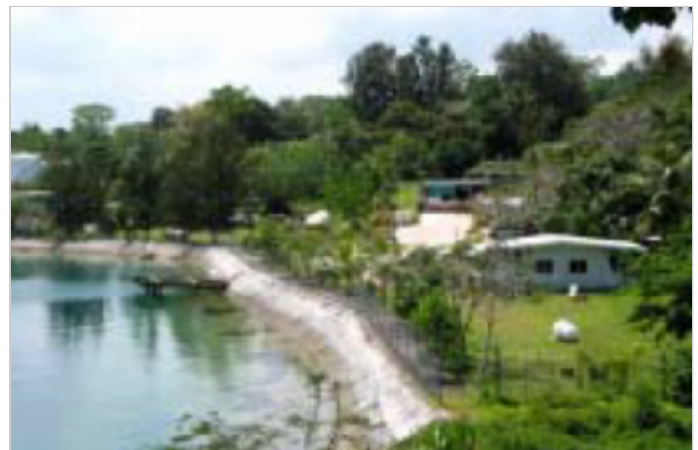
General View of Boral Gas Depot
