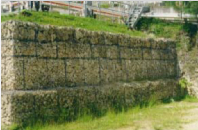
Corner view of wall pre earthquake
