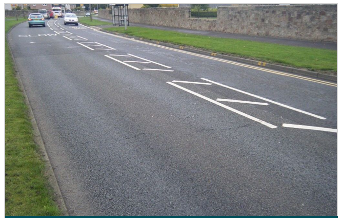
Road Mesh was installed in two different overlay thicknesses
