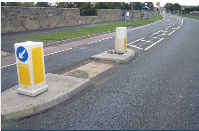
The trial site uses both Road Mesh™ and geogrid
