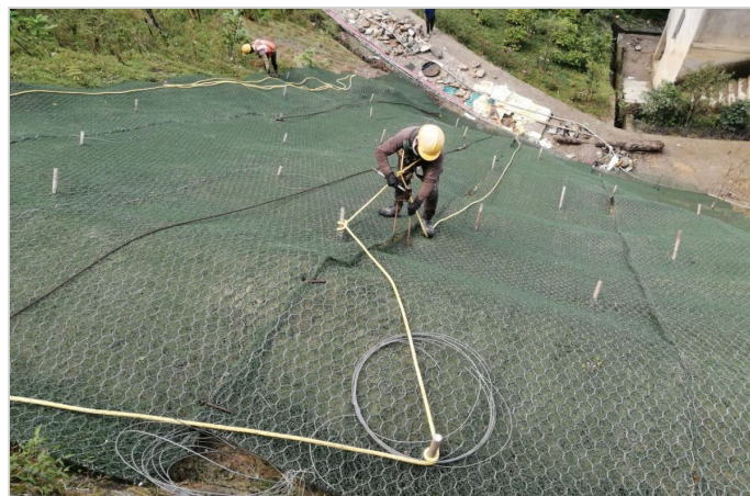
Figure 4-Protected slope during installation of Macmat R
