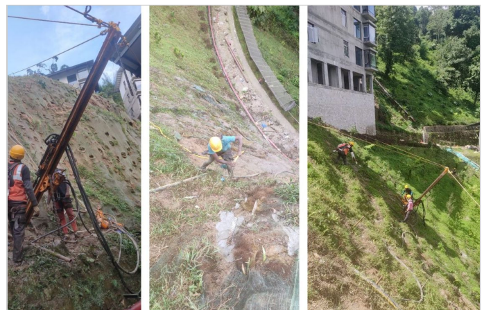
Figure 2-Installation of nails
