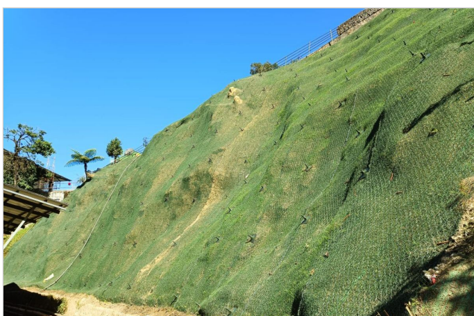
Figure 5-Slope after the installation
