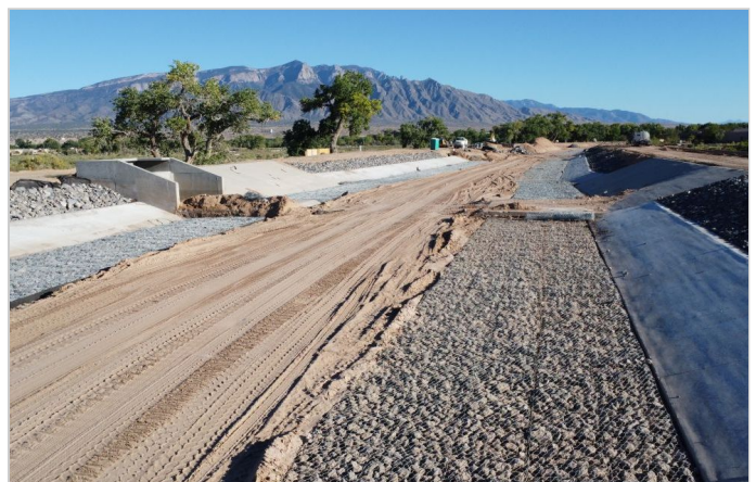
Lower Bank Stabilization
