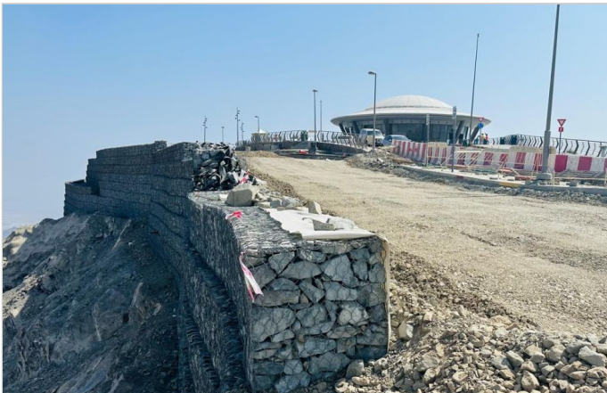
Terramesh wall in progress
