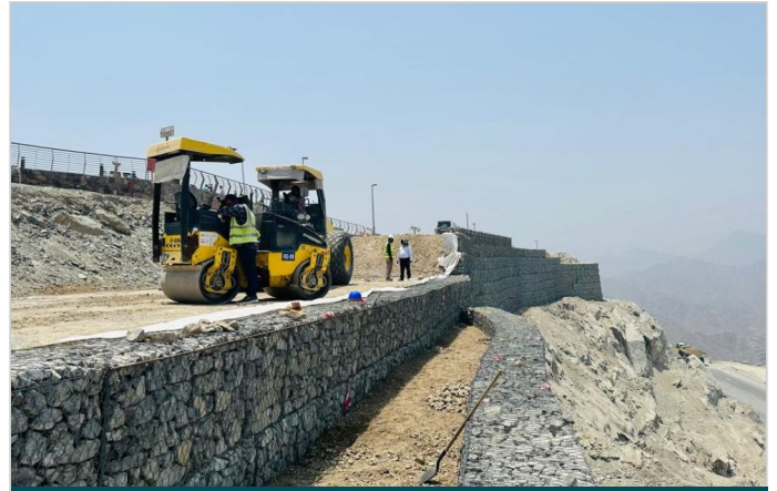
Terramesh wall in progress
