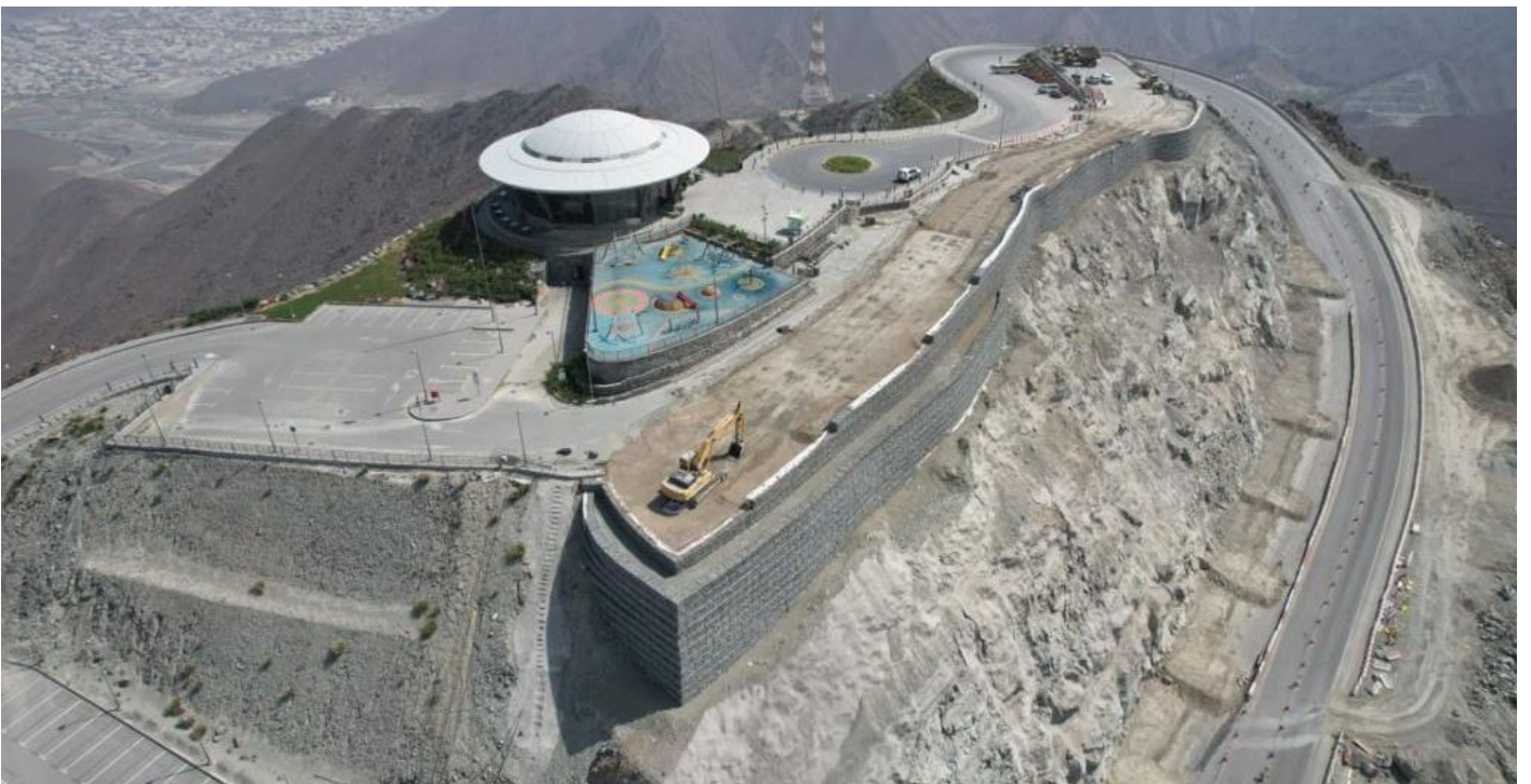
Completed: aerial view of Terramesh wall at parking area
