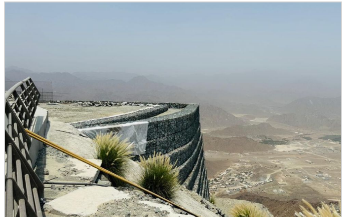
Completed: side view of Terramesh wall
