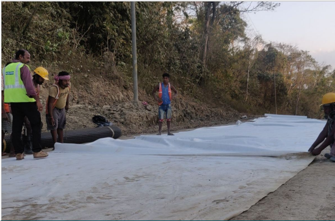
Photo 3: During construction - laying of MacTex
