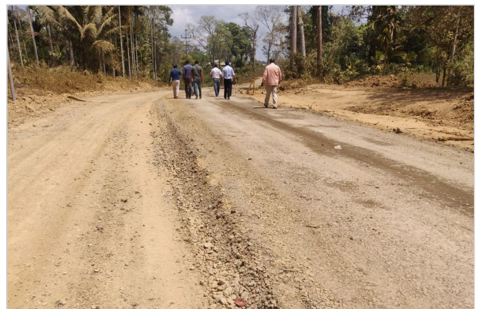
Photo 2: Site preparation before construction
