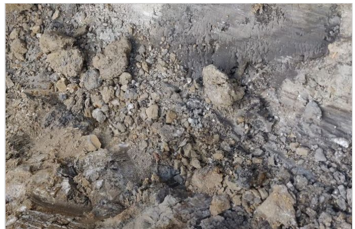
Photo 1: Condition of soil at site
