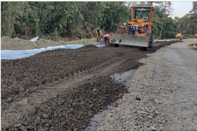
Photo 5: Layer of 60 mm, crushed aggregate over MacGrid
