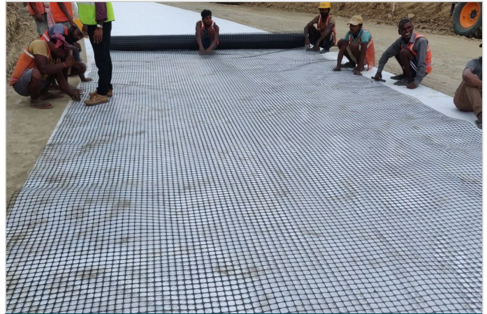
Photo 4: During construction - unrolling of MacGrid EG over MacTex
