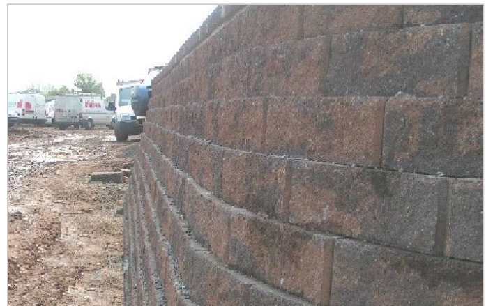
Post construction of MacWall
