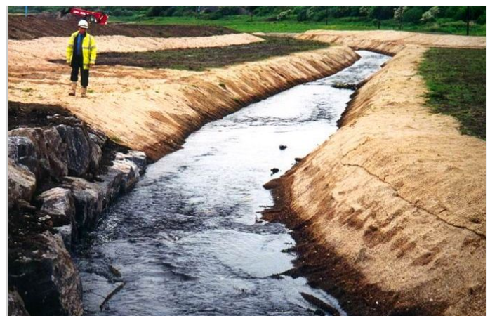
Biomac secured to the new channel bank flood berms
