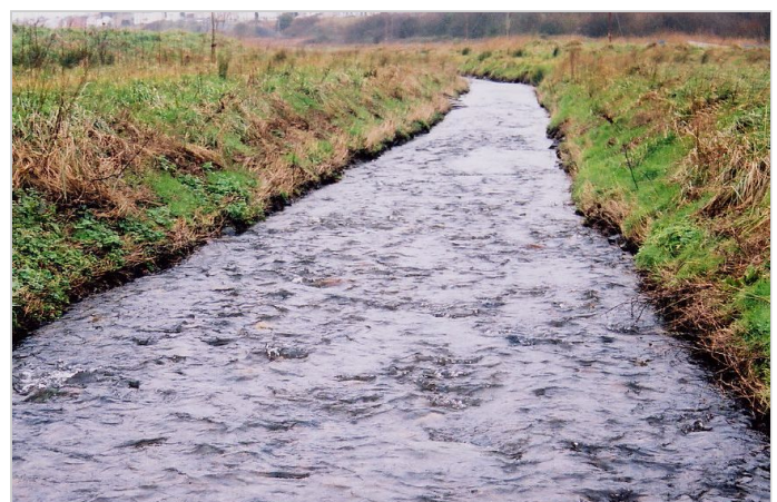
18 months after construction, vegetation has established well
