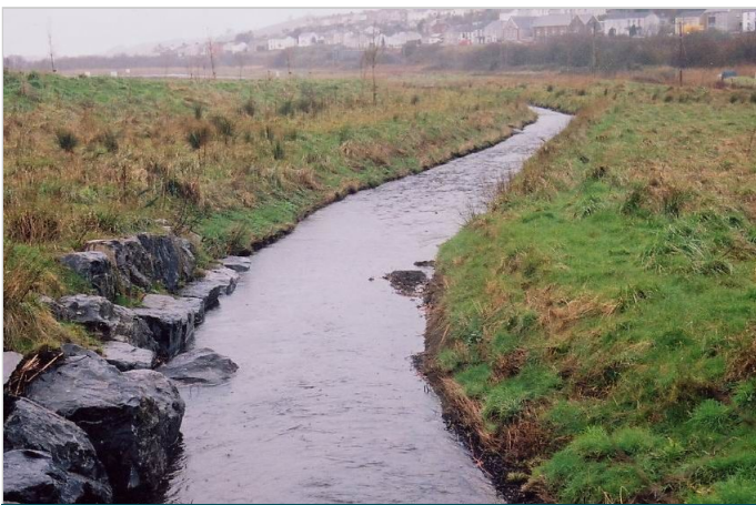
Blockstone & Reno mattresses protecting outside bends
