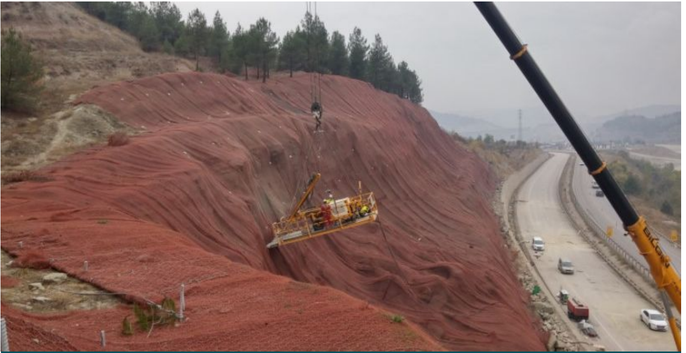
Macmat HS, Rock Bolt and Diagonal Rope Application
