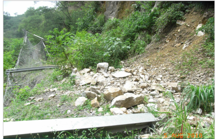
Rockfall Debris Impact at Base of Post
