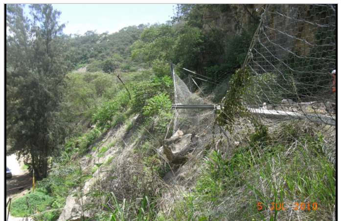
Rockfall Debris Impact on Fence
