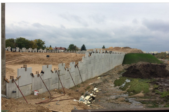
The panels were stored on previously completed MacRes Wall
